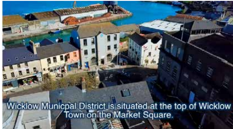
Wicklow Municipal District Offices on Market Square
